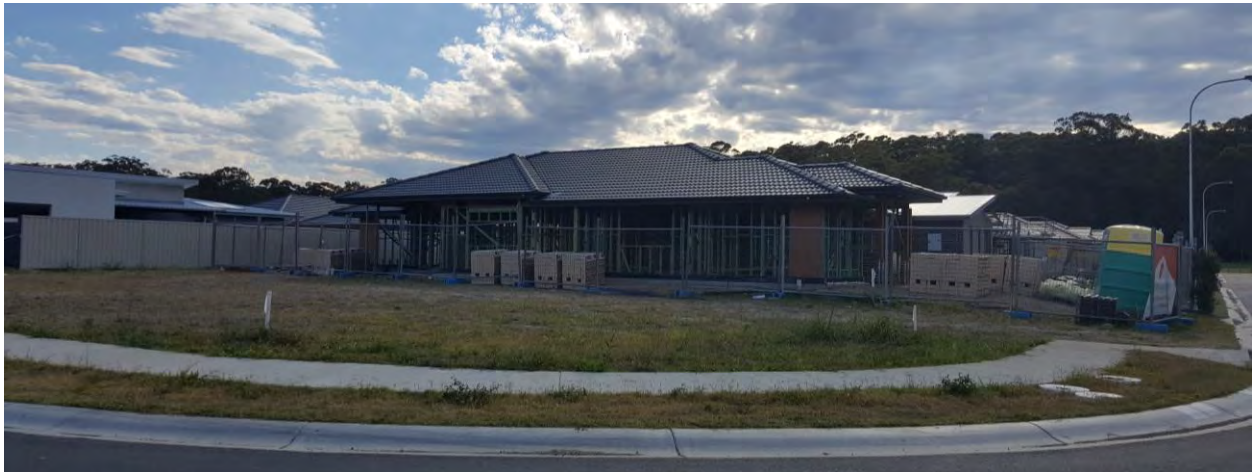
Detached housing construction at North Sandy Beach
